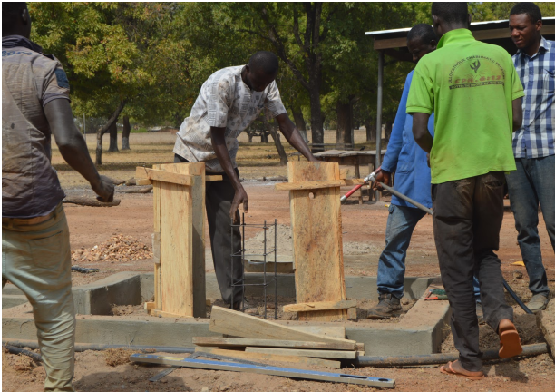
Setting up distribution point mold
