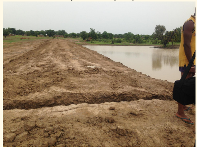
Trench constructed for the dam
