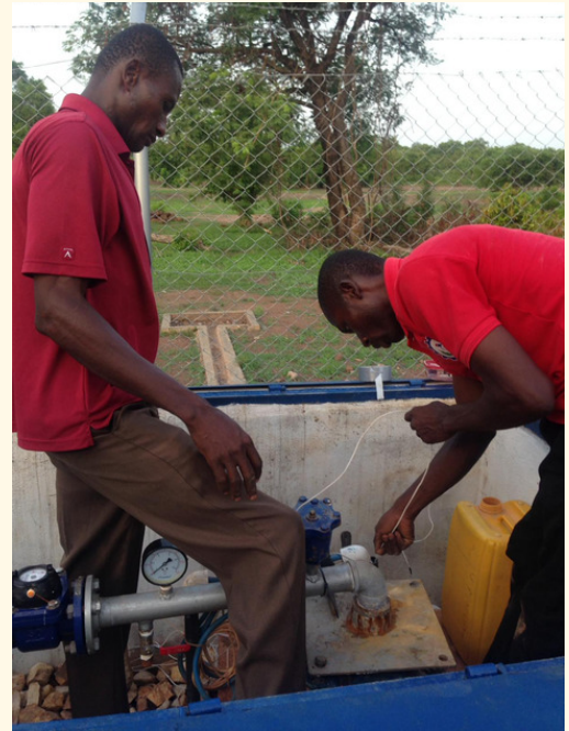
Installation of the water level sensor
