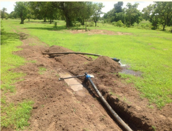
New valve for the chlorine pump being added
