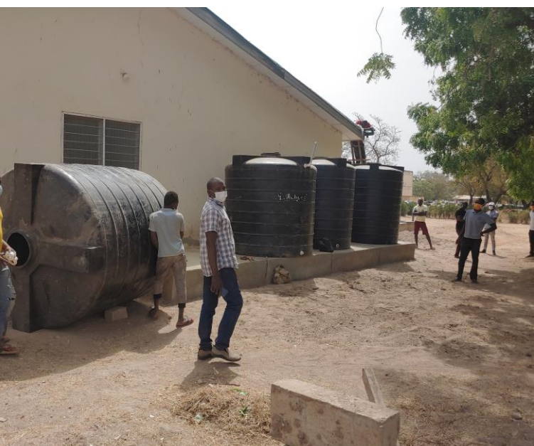
Tanks to which gutters and piping were routed
