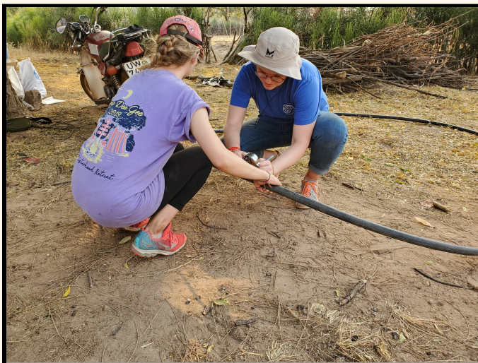
Mary and Jennifer measuring out and marking piping for the micro irrigation system which will utilize rainwater collected from a portion of the school dining hall.
